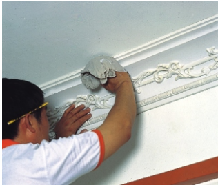
10.Wipe off excess filler.
