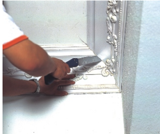
6.Adjust the joint for perfect match.
