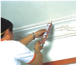
8.Apply filler to fill up gaps.
