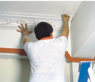
1.Make marking on cornices for corner joint.
