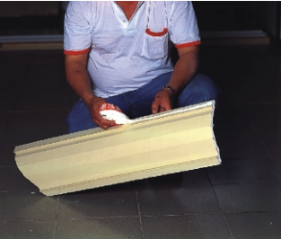
4.Apply adhesive along the edges at the back of cornices as well as to the mating surfaces for joints.
