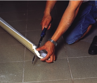
3.Saw at the marked point of the cornice.
