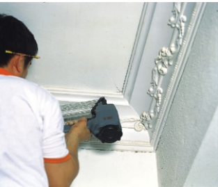
7.Ensure proper alignment on joints before nailing.
