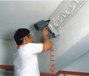
5.Using Pressure gun for nailing.
