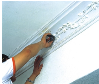
9.Use sand paper to smooth the surface.
